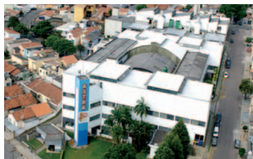
ASTRA I - INJECTION FACILITY
