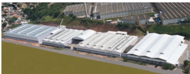
ASTRA VII - ALUMINIUM AND FIBERGLASS FACILITY
